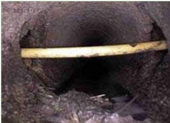
*Example of a problematic cross bore of a gas pipeline through a sewer line*
