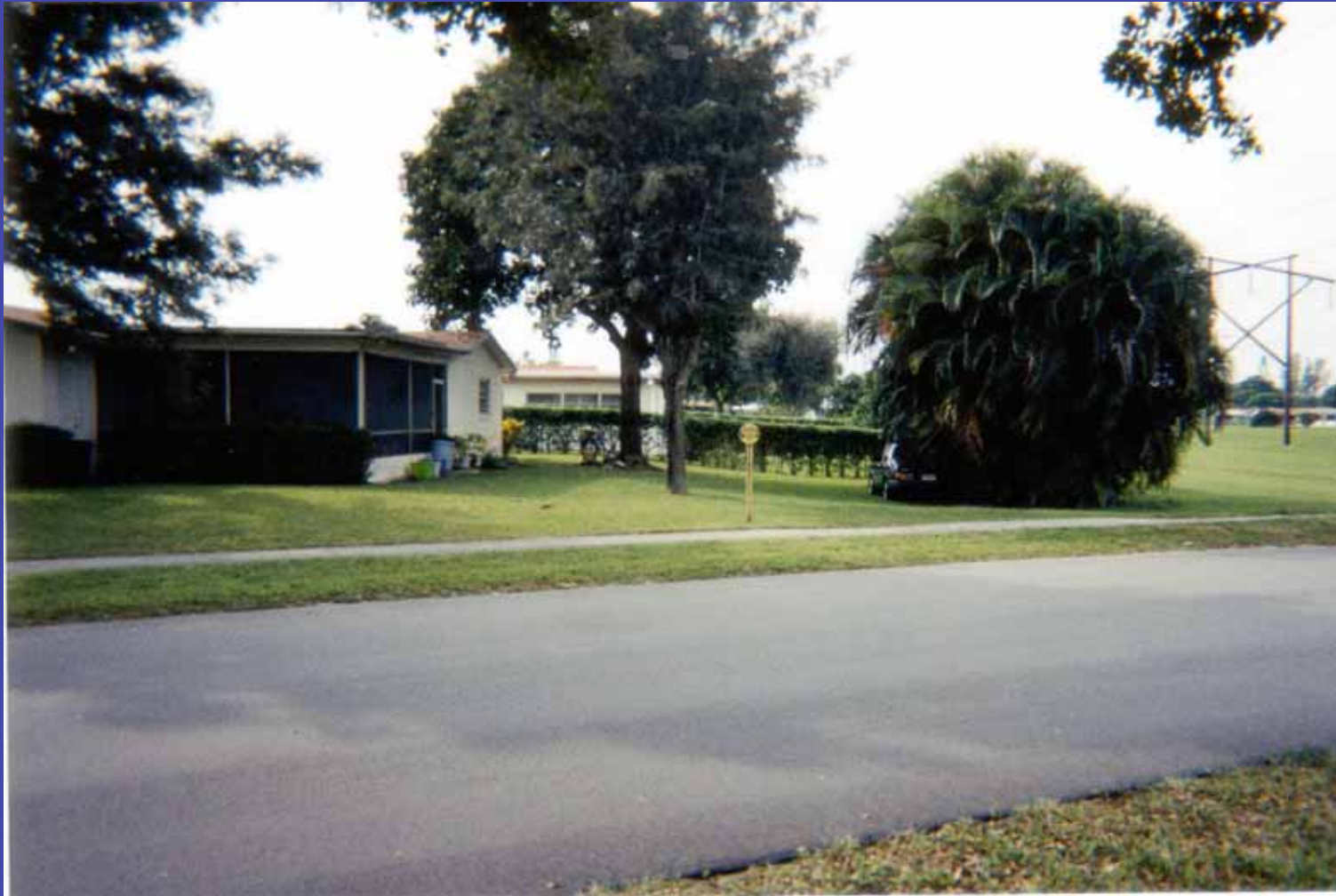
Everglades Pipeline Crossing NW 23 St. (Looking South)
