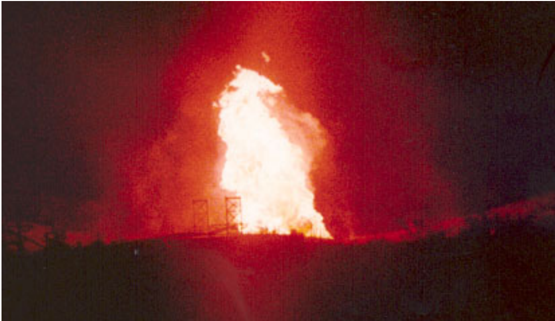
Figure 5. Post-rupture fire. At lower left of fireball can be seen the 85-foot-tall support structures for the pipeline suspension bridges.
